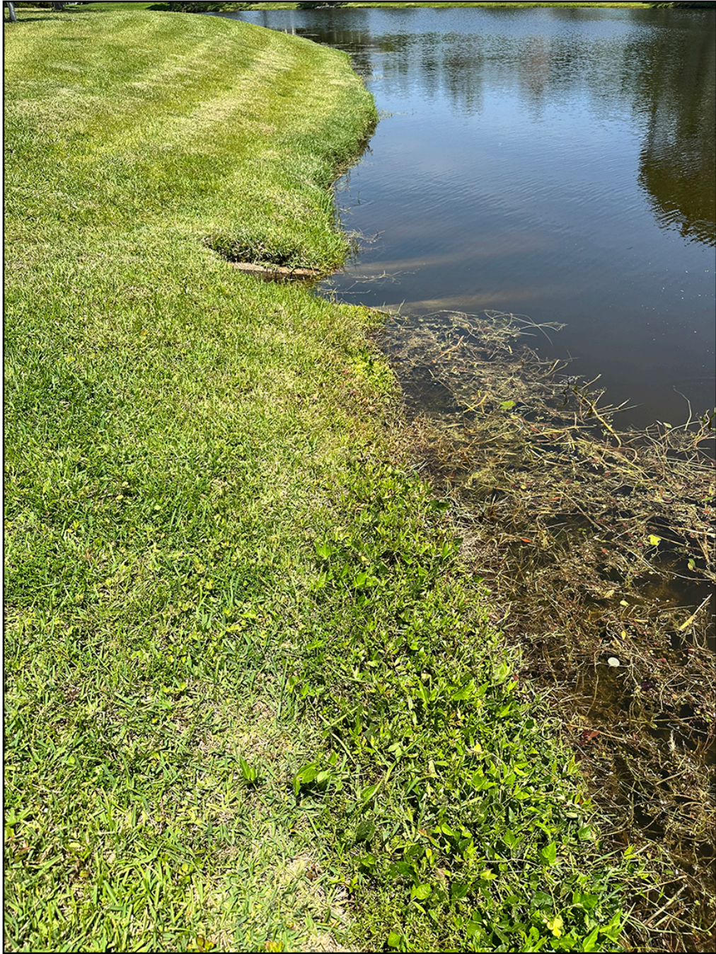
Figure No. 2: Pond #6 Lake bank area exhibiting slope issues caused by erosion.
