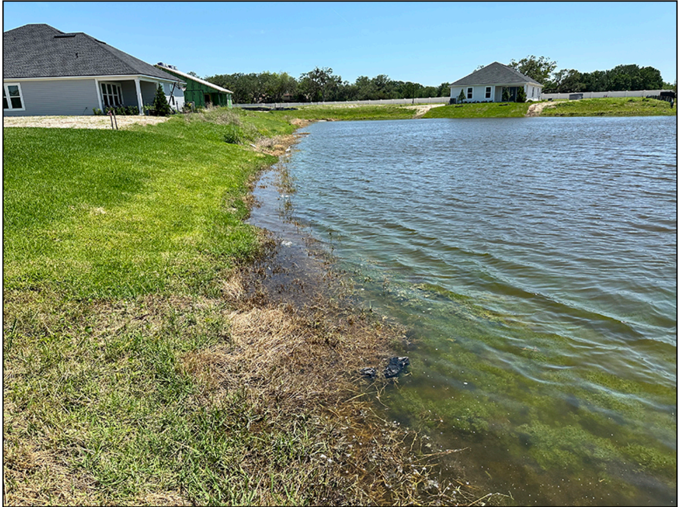
Figure No. 6.- Pond #11 various levels of erosion effects along the entire embankment.
